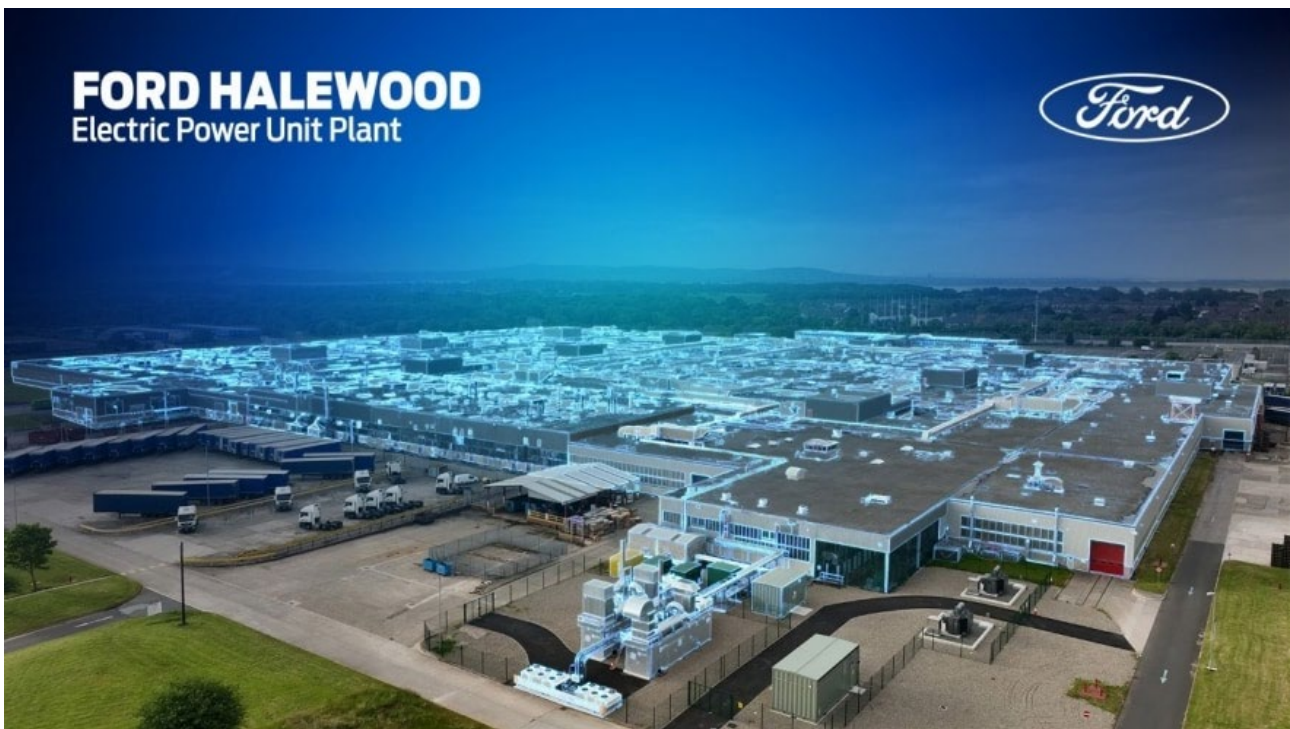
Figure 2: Ford's Halewood facility in the UK (source: www.ford.com ).
