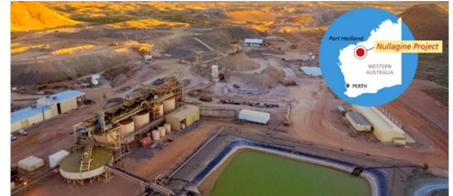
Aerial image of Golden Eagle Plant
