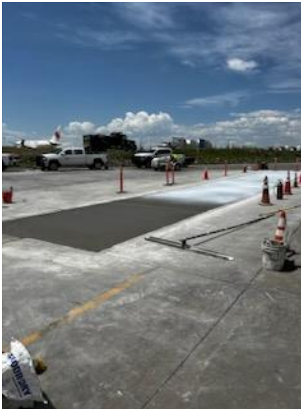
Figure 1. Concrete being replaced in full depth slab
