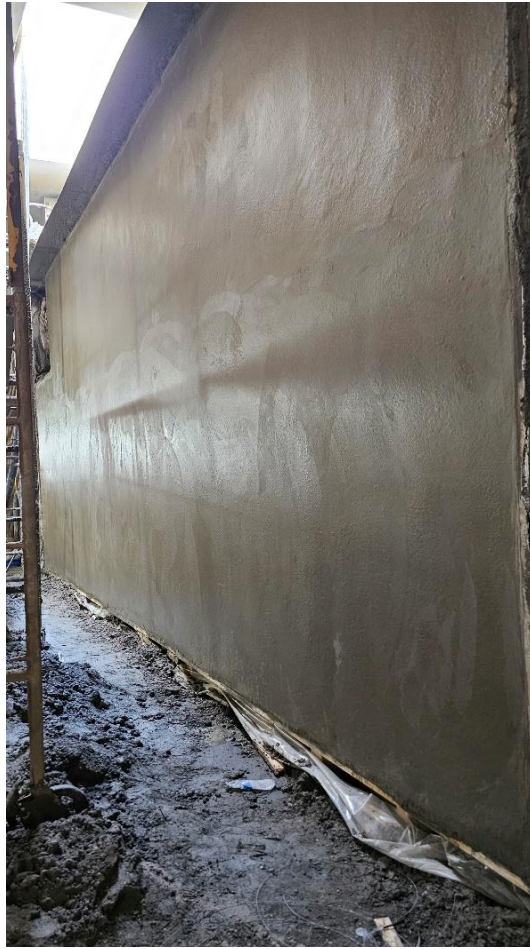
Figure 10. Completed wall showing very smooth finish
