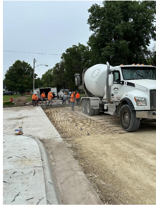
Figure 7. Concrete pavement being poured
