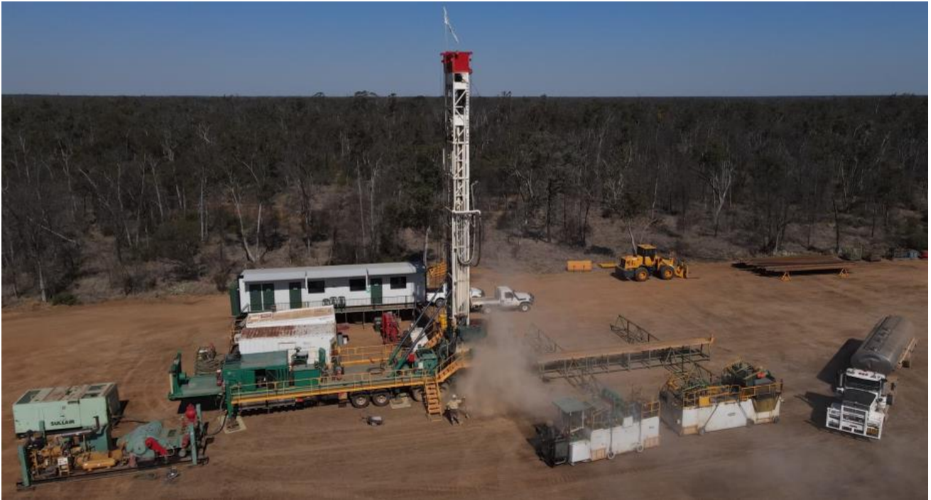
Water well drilling at Daydream-2 wellsite
