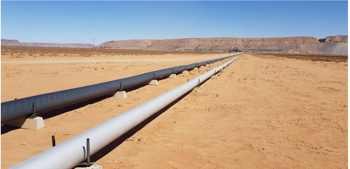
Figure 11: Example of overland pipes the concept planned for Kasiya (Source: Paterson & Cooke)
