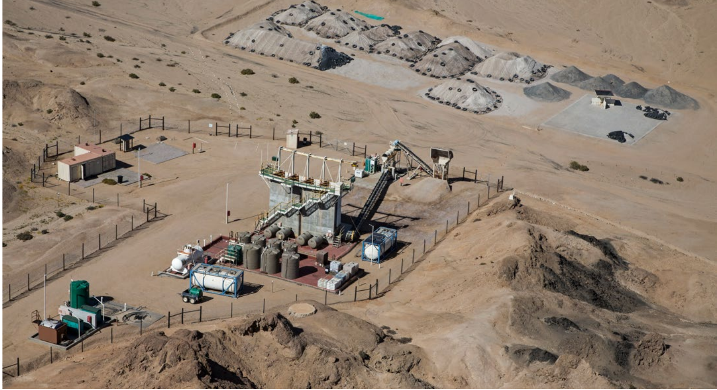
The Heap Leach Demonstration Plant for the Etango Uranium Project within the Namib Desert
