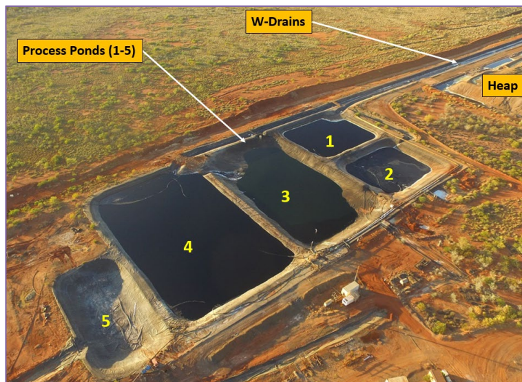
Figure 3: Process ponds 1 to 5 and W-drains cleaned and certified
