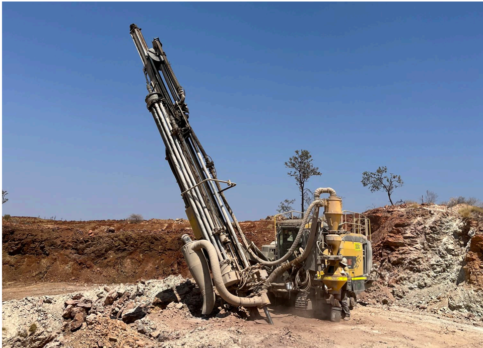
Figure 2: Drilling underway at the Blue Bar Open Pit (Haoma JV Project)
