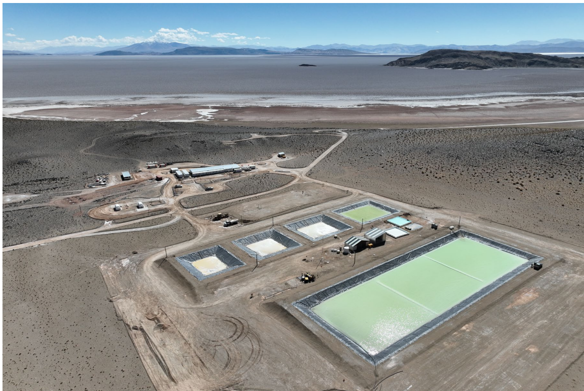
Figure 14: Pilot Plant at HMW
