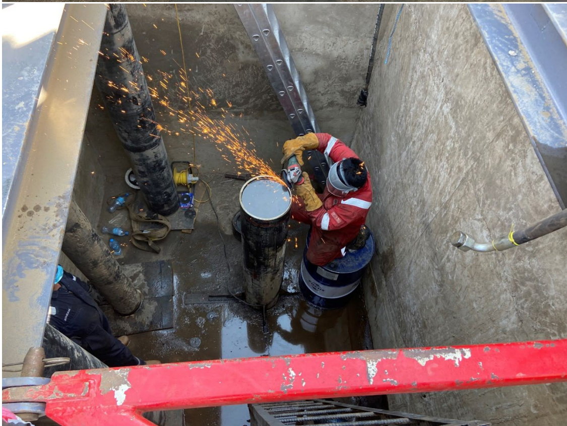
Figure 1. a) Mbelele-1 Wellsite and b) preparing for wellhead / BOP installation at Mbelele-1
