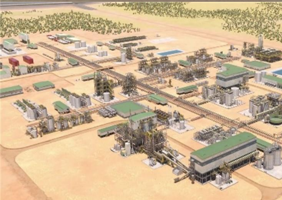
Sulphation & Concentrate Handling Buildings
