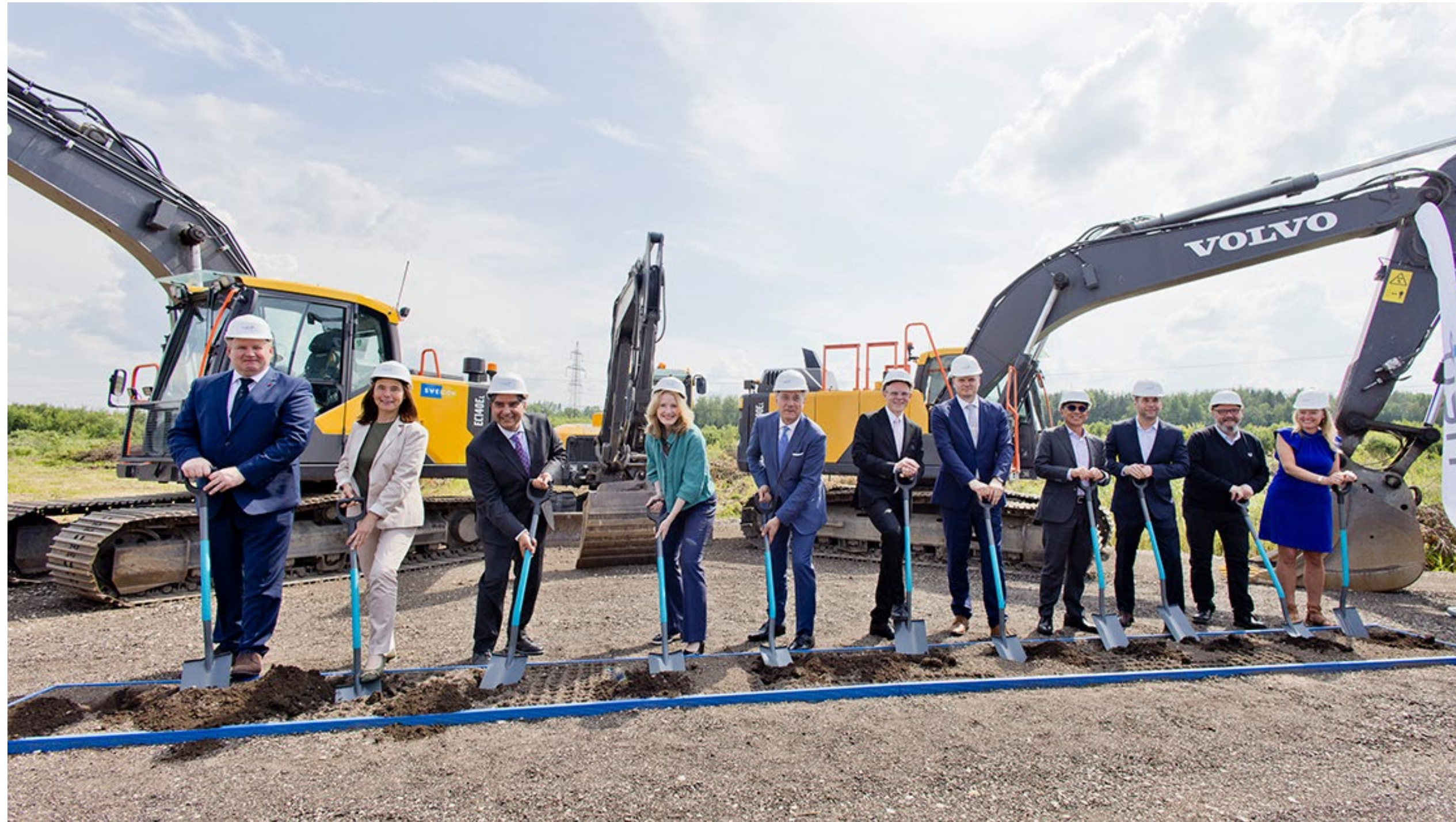
Picture: Groundbreaking ceremony for Neo's sintered rare earth magnet manufacturing facility in Estonia
