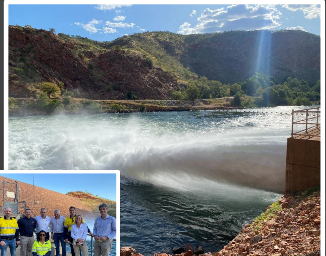
Figure: Members of the Boab and Horizon Power teams on site at the Ord-Hydro Power station.
