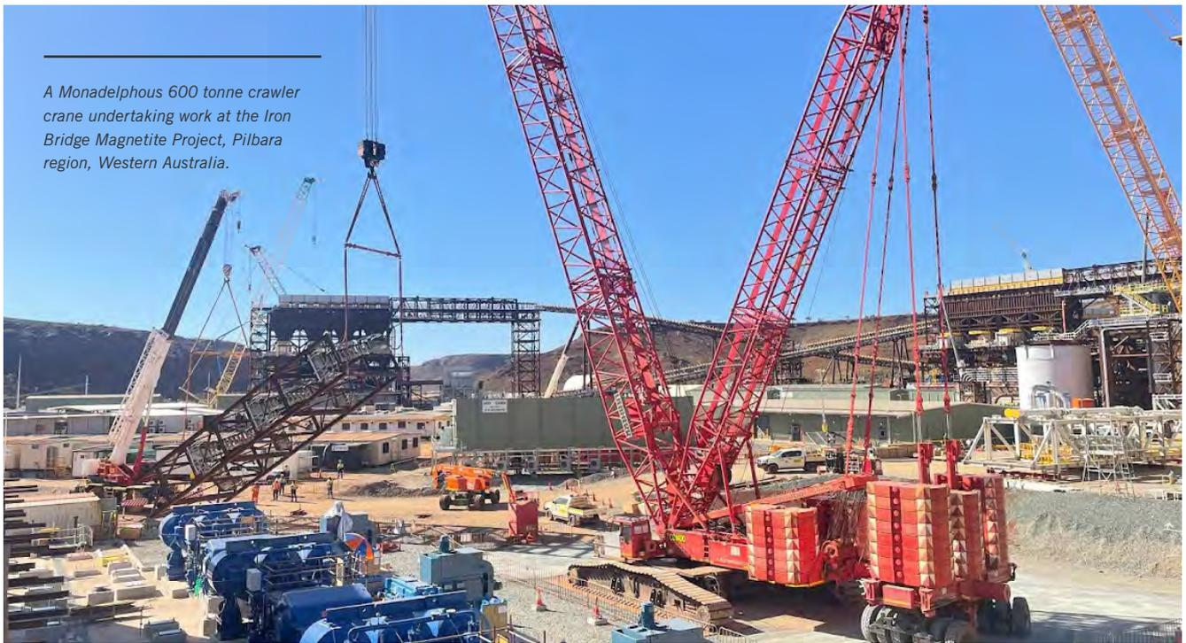
*A Monadelphous 600 tonne crawler crane undertaking work at the Iron Bridge Magnetite Project, Pilbara region, Western Australia.*
