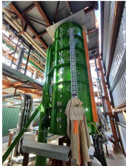
Furnace installation completed and operationally tested
