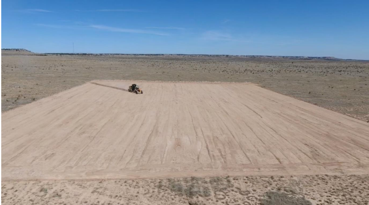
Figure 2: Site preparation construction works progressing at the Voyager facility site
