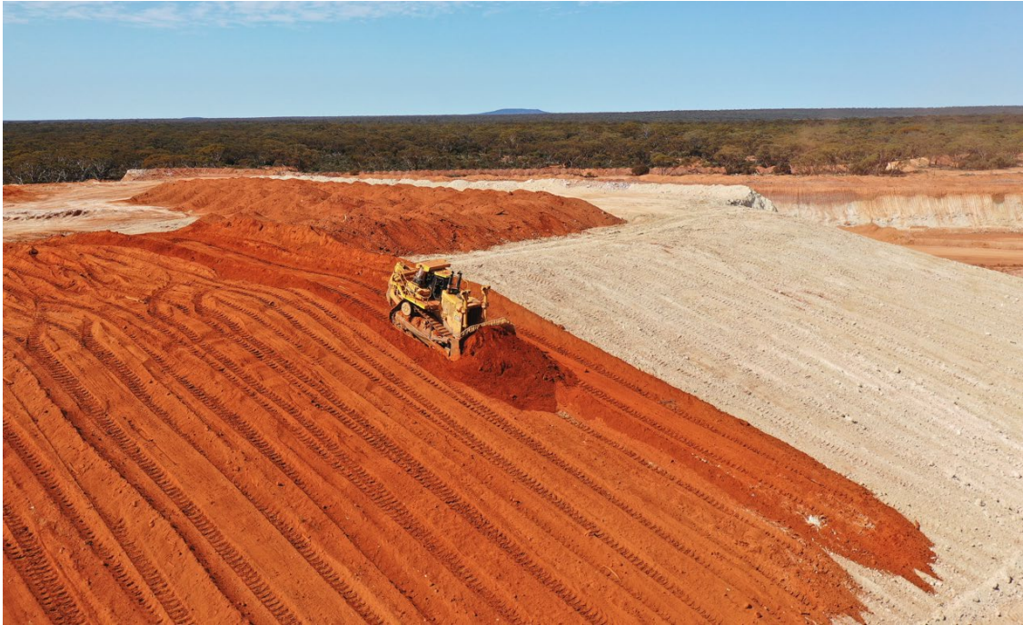
Figure 1: Dozer spreading topsoil on the Lost Dog waste dump on 25 August 2023
