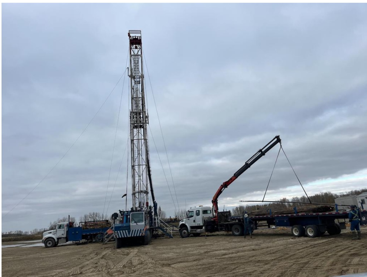
Figure 1 – Service rig conducting workover operations at Rex-4
