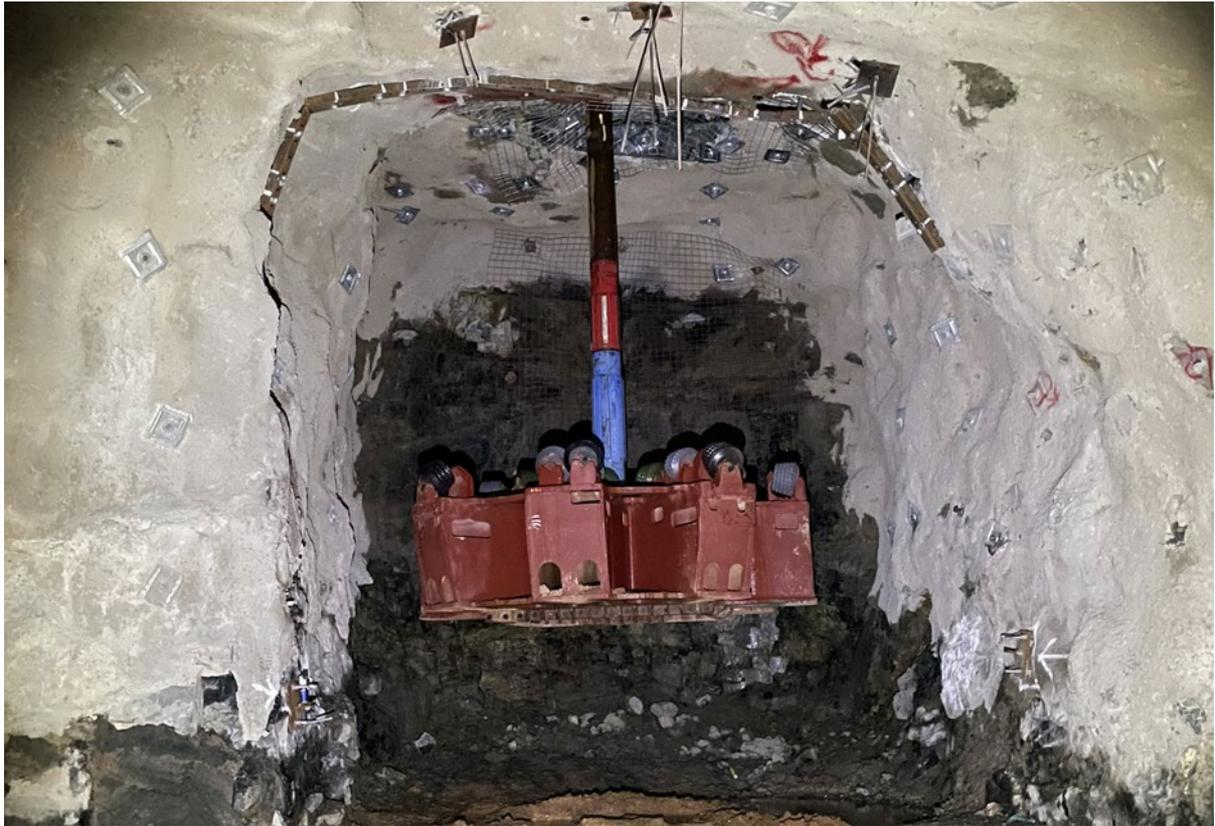
*Figure 5 - Reamer installed and ready to commence back-reaming the 4.5m diameter return air raise*
