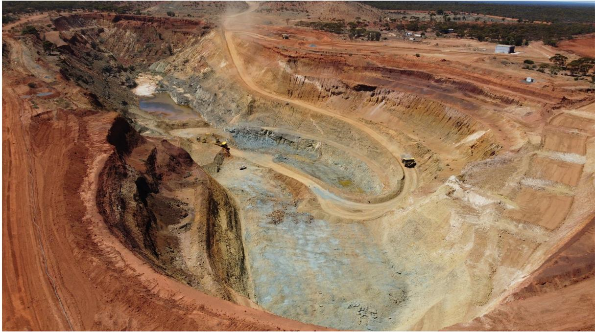
*Figure 2 - View of Sand King looking north showing cut back commenced in the southern half of the open pit*
