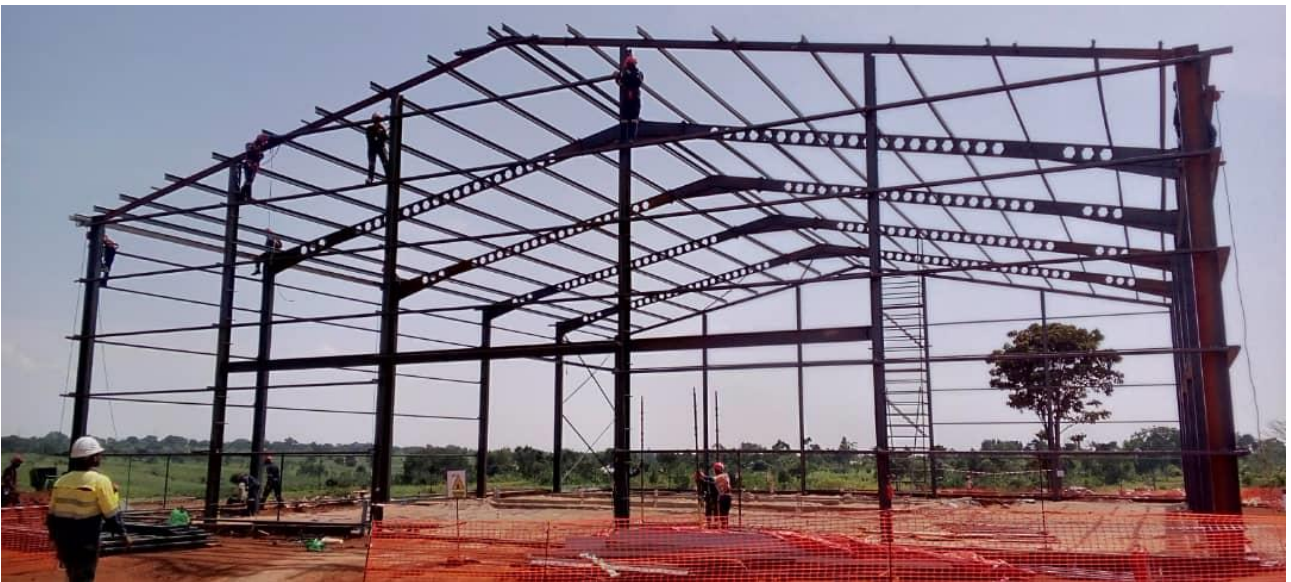
Figure 9: Makuutu Technical Facility frame structure erected.
