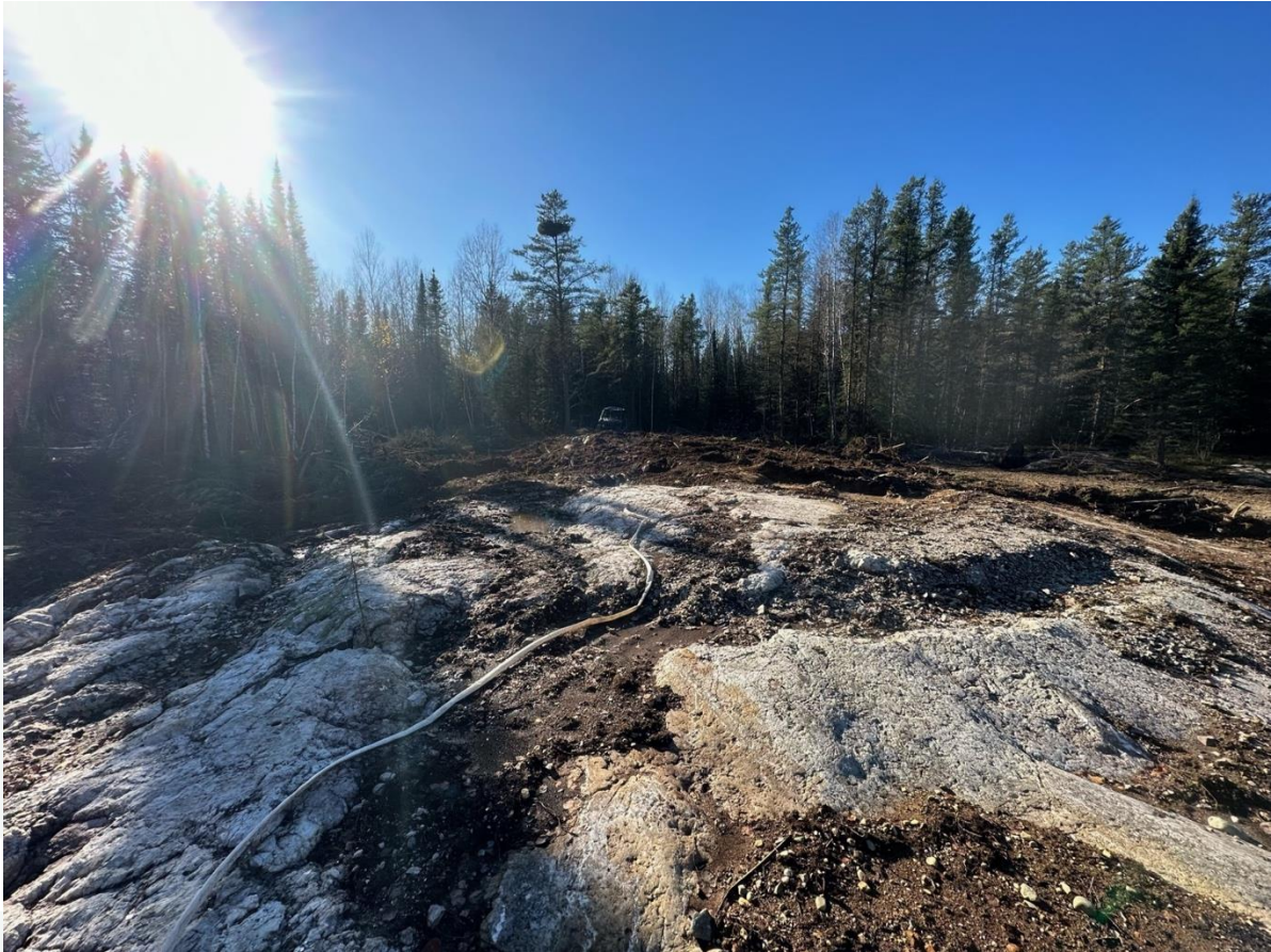
Figure 2: Additional drill pads being prepared at Koshman.
