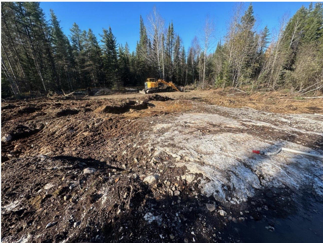
Figure 1: Stripping and washing ongoing at Koshman.
