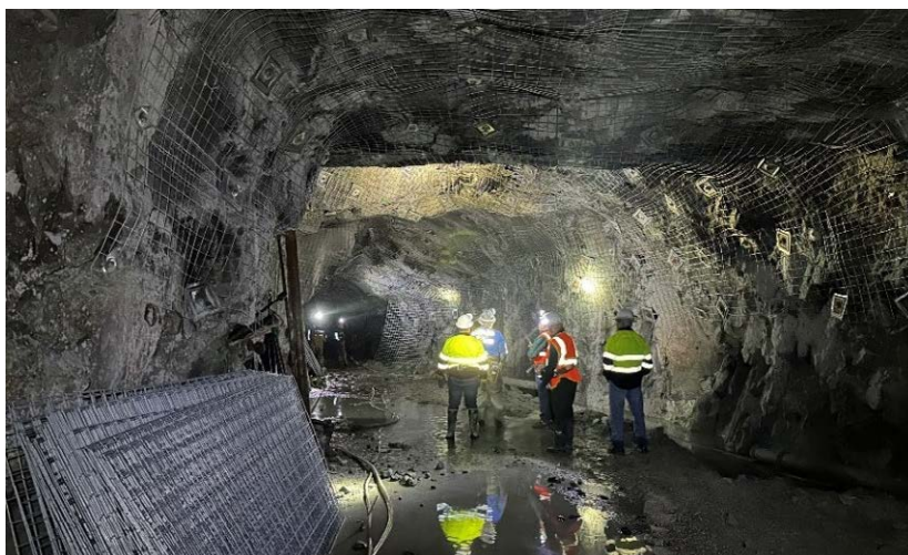
Underground mine refurbishment in progress
