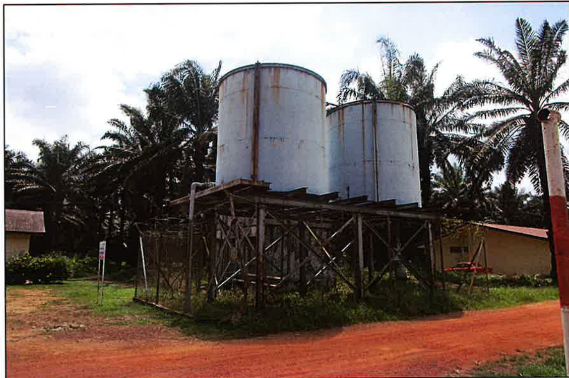
VIEW OF WATER TANK
