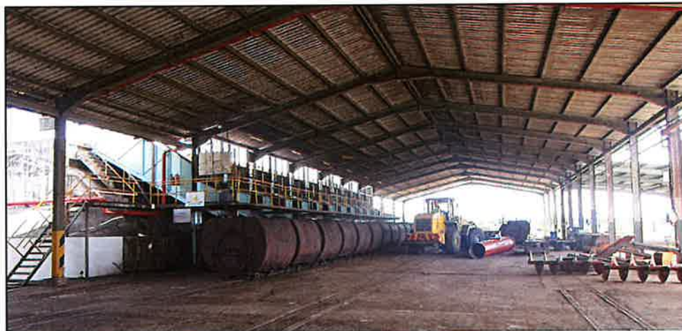
VIEW OF TRANSFER CARRIAGE AND LOADING RAMP
