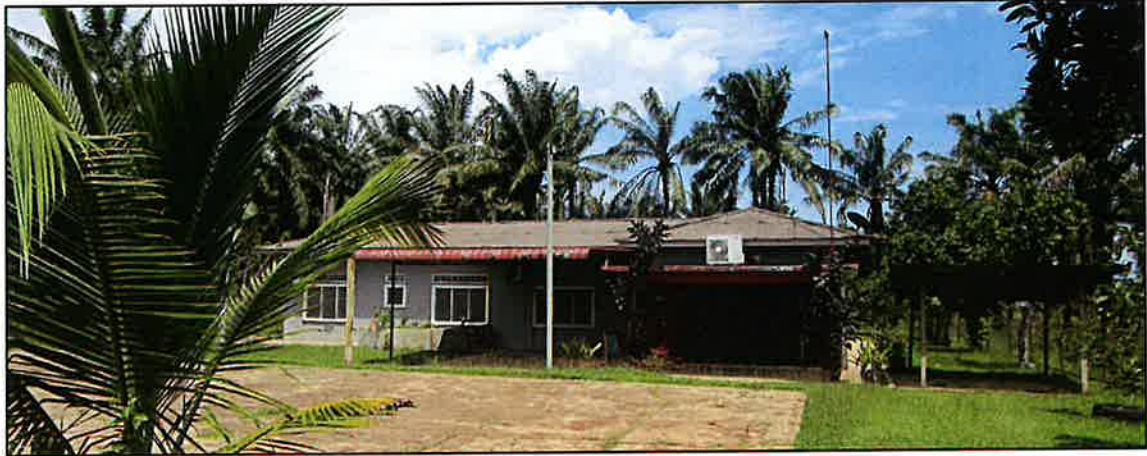
VIEW OF MILL MANAGER'S BUNGALOW
