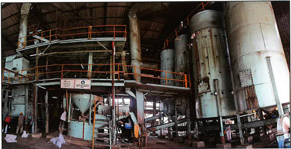
VIEW OF KERNEL PLANT
