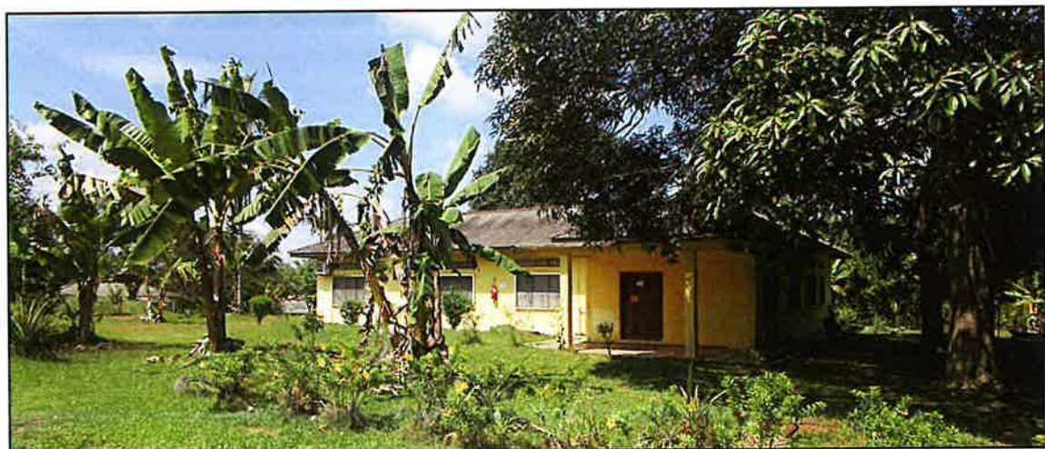
VIEW OF THE MANAGER'S BUNGALOW
