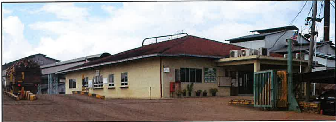
VIEW OF THE OFFICE BUILDING
