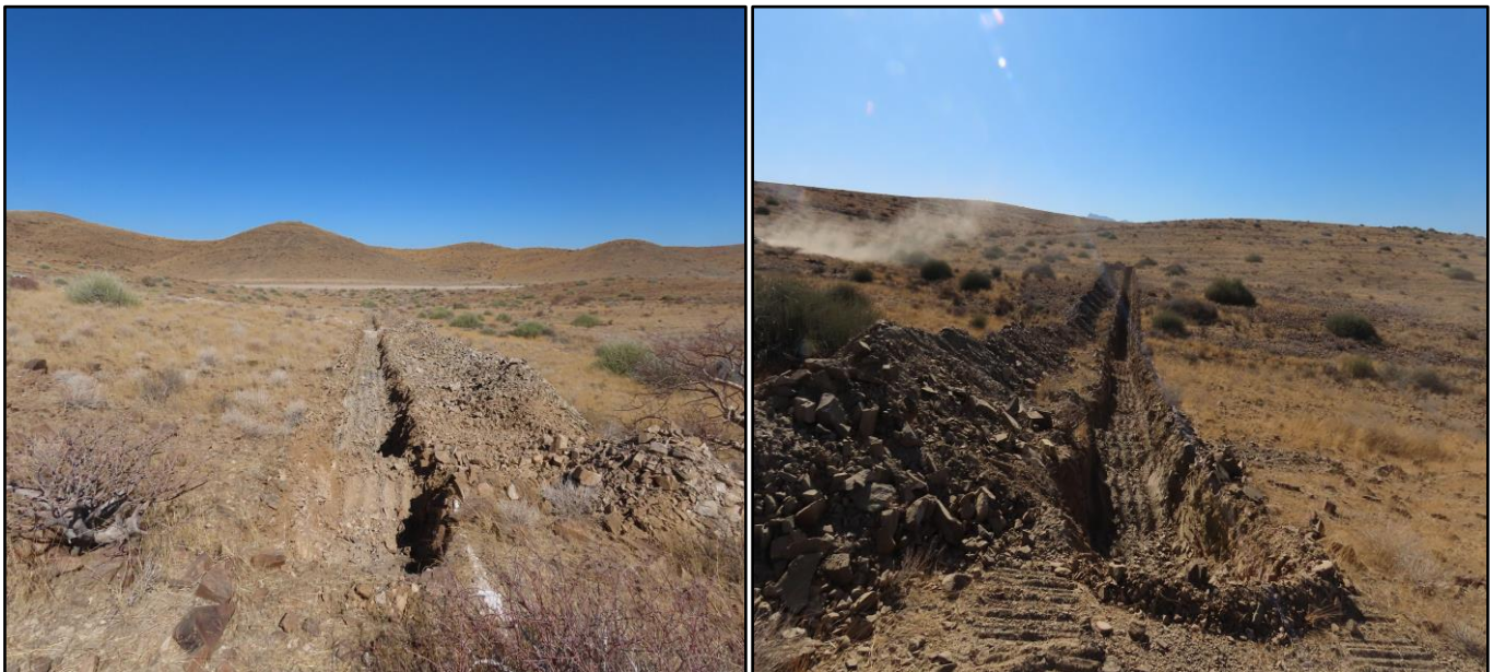
Figure 11 and 12: Progress on trenches pOPT_20 and pOPT_19.
