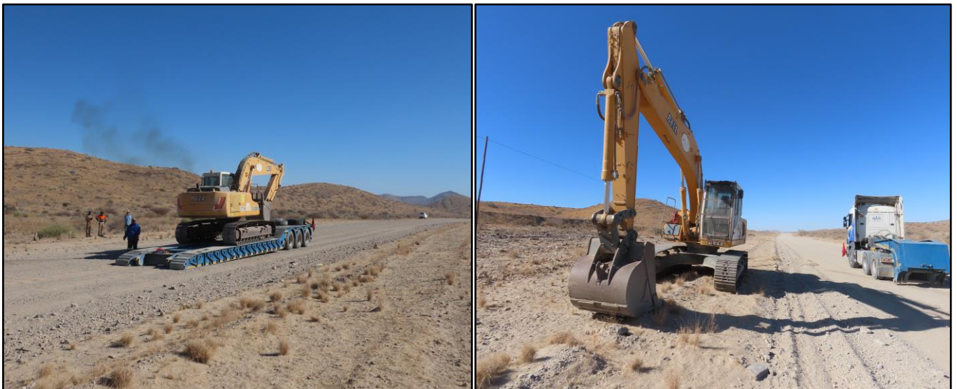
Figure 3 and 4: Excavator being offloaded on EPL 7345.
