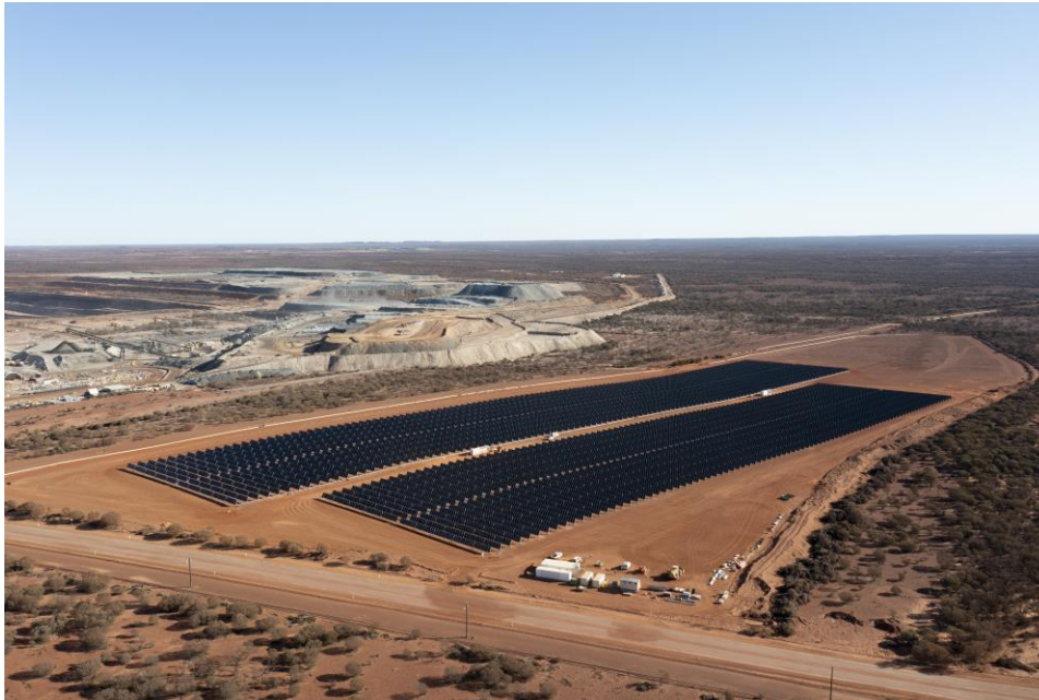
Figure 1: 9MW solar farm at Duketon South
