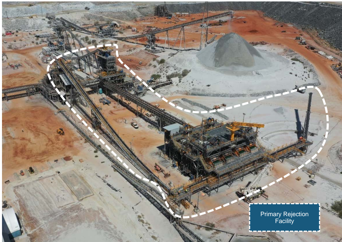
Figure 1: P680 Primary Rejection facility
