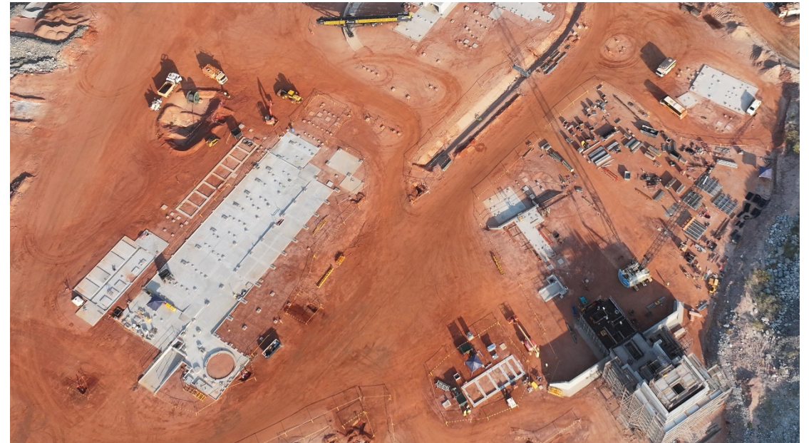
Crushing and ore sorting facility concrete poured
