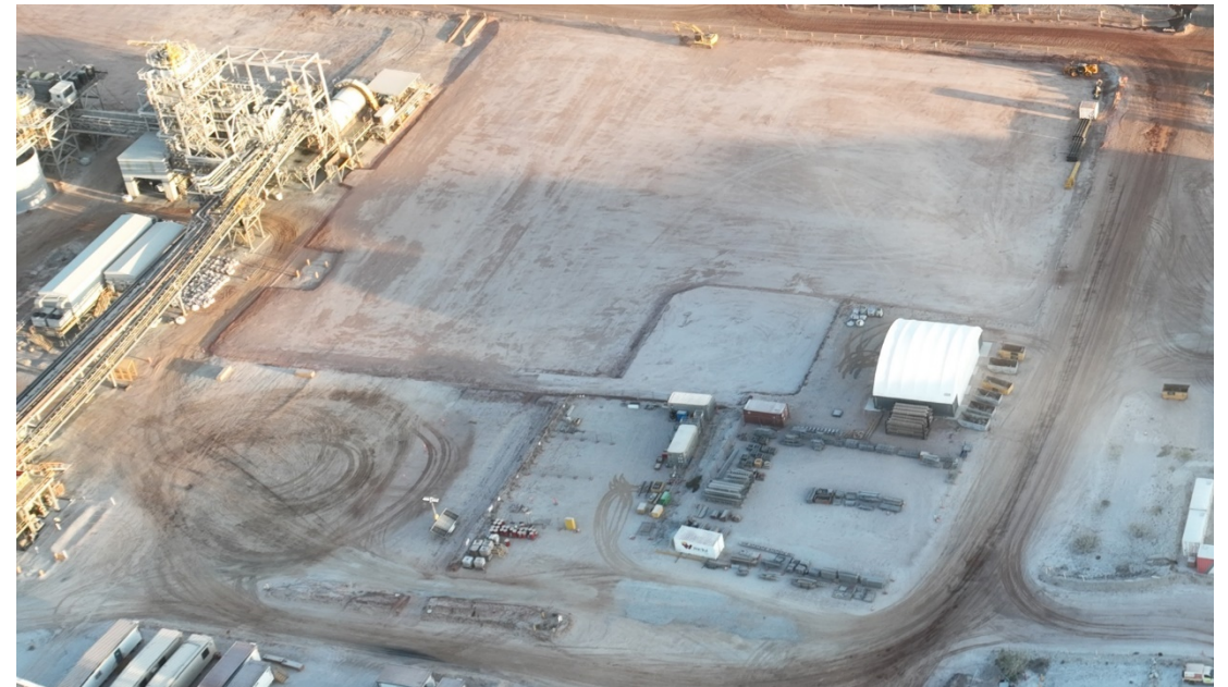
P1000 earthworks commenced
