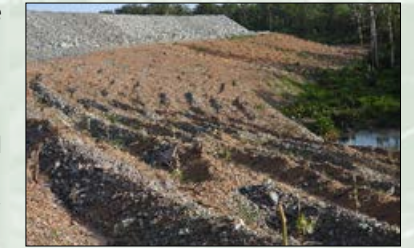
Figure 34 | Rehabilitated batter on waste dump
