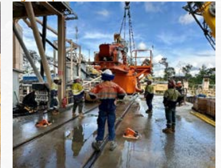
Figure 6 | Okvau Maintenance Personnel
