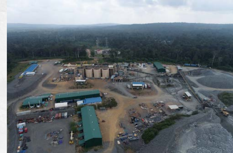
Figure 2 | Okvau Gold Mine infrastructure
