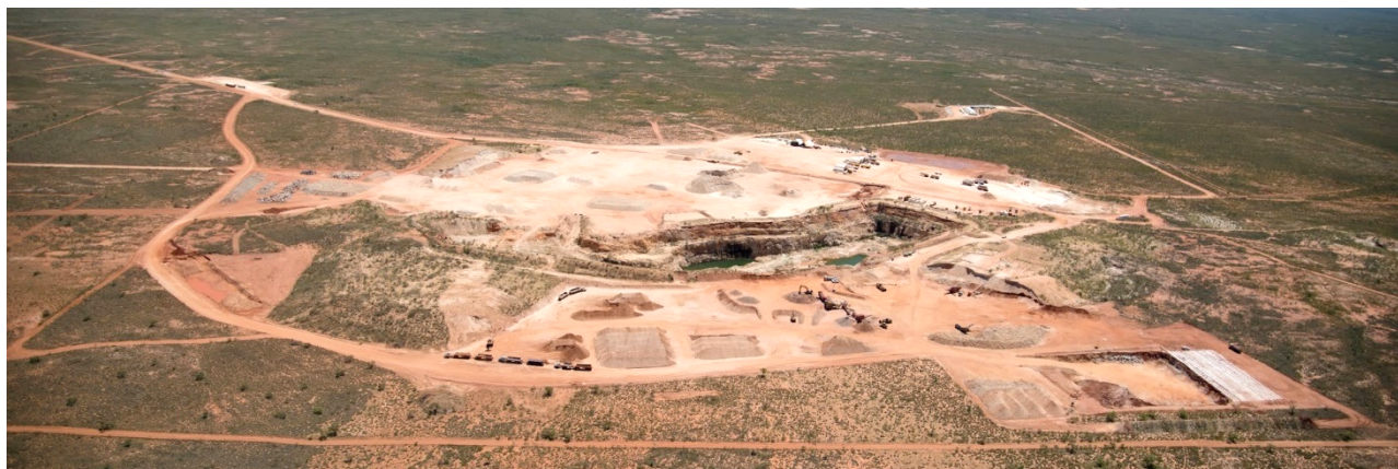
Plate 1: Pippingarra Quarry and Associated Infrastructure
