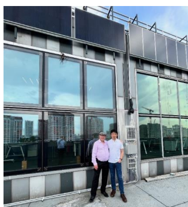
Second Generation ClearVuePV vision glass testing IGU's and spandrel panel units (above the glazing) installed and being prepared for commencement of BCA testing.
