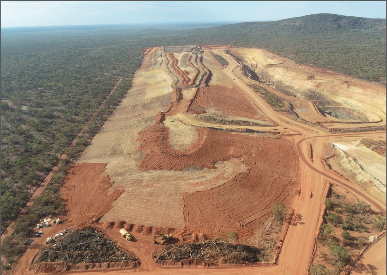
Figure 5: Topsoil spreading as part of ongoing rehab at Die Hardy pit (Marda)
