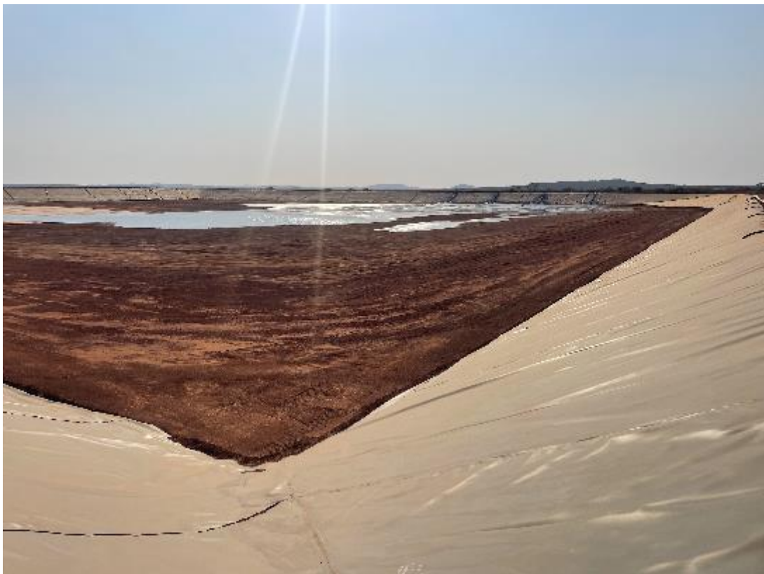
Figure 11 – Abra TSF Stage 1B (photo 23 October 2023).
