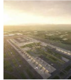
Multiplex Western Sydney International Airport - Heyday Over $100m
