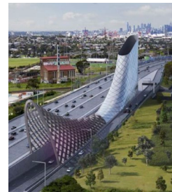
Westgate Tunnel Switchboards – Trivantage Manufacturing Over $10m
