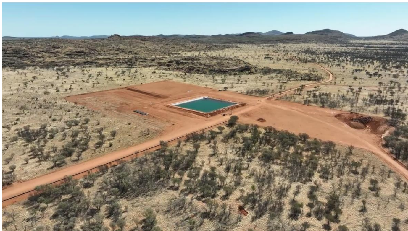
Figure 5: Completed site raw water storage dam, September 2023
