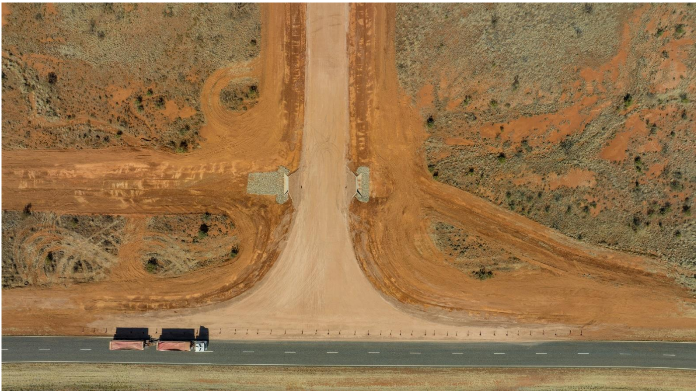
Figure 4: Aerial view of the Nolans Project site access temporary intersection with Stuart Highway, September 2023
