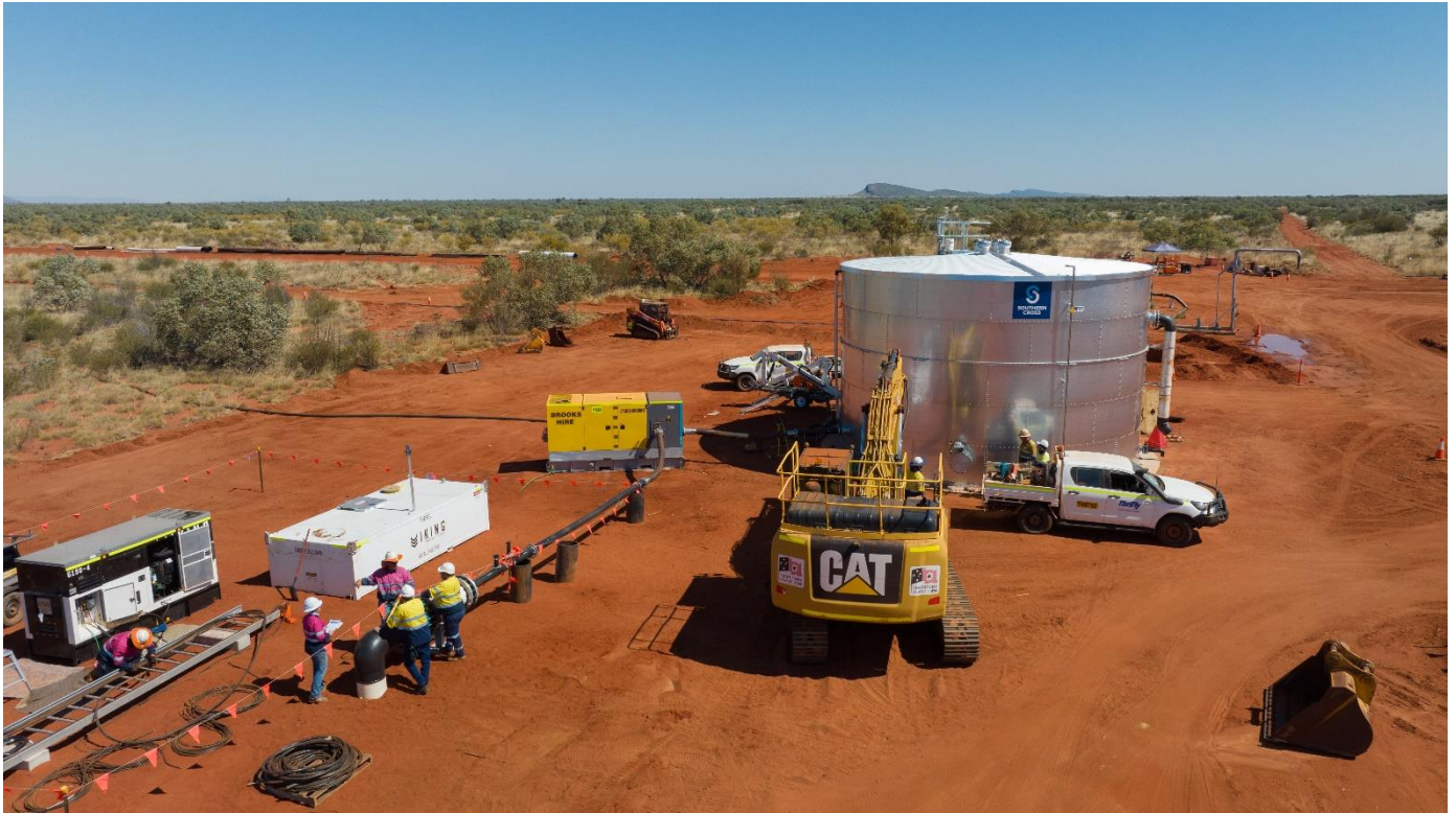
Figure 3: Water storage tank and pump infrastructure installation, August 2023
