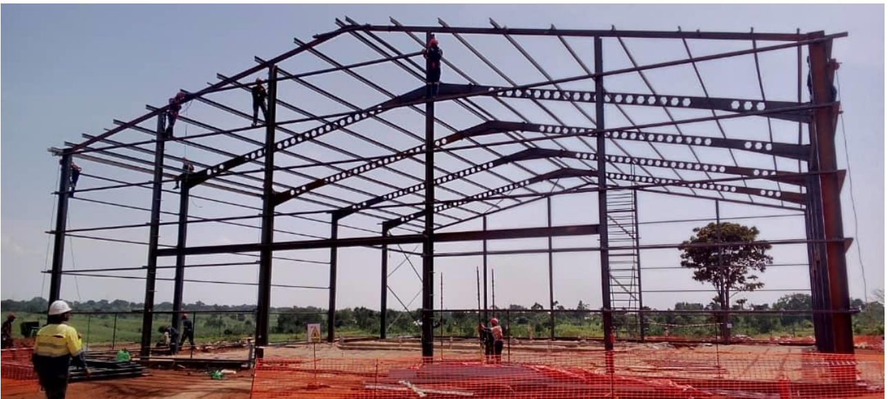
Figure 3: Makuutu Technical Facility frame structure erected.
