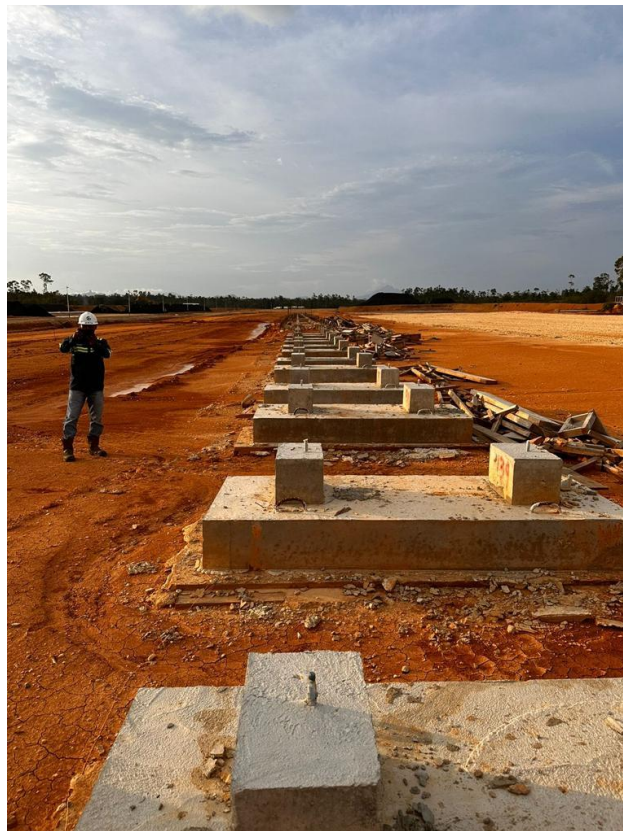
Conveyor Structure foundation works
