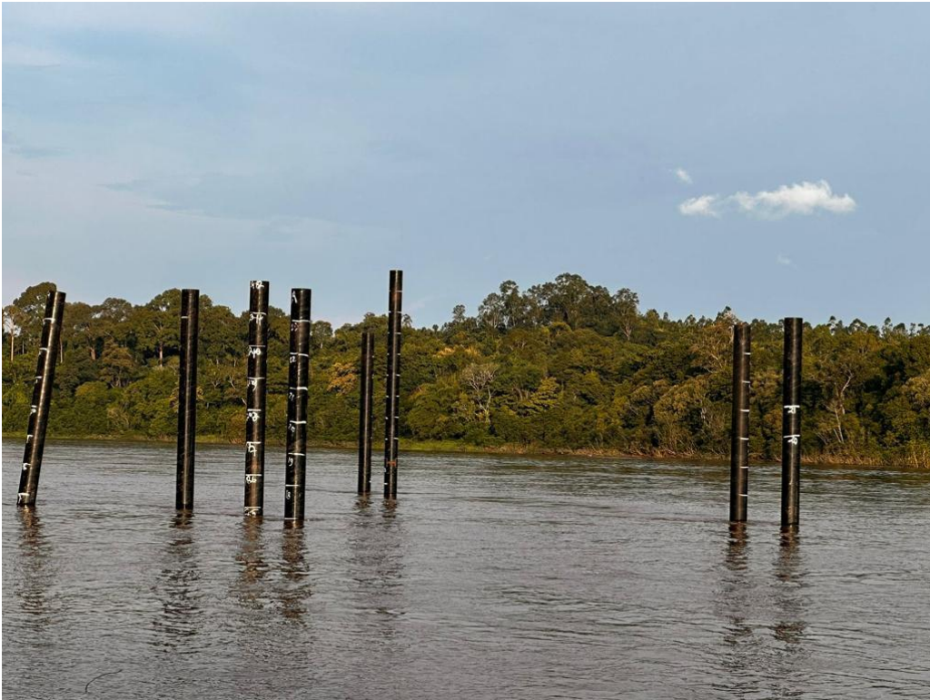
Piling works at jetty
