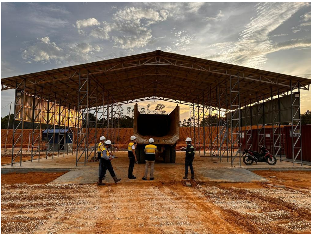
Truck maintenance workshop
