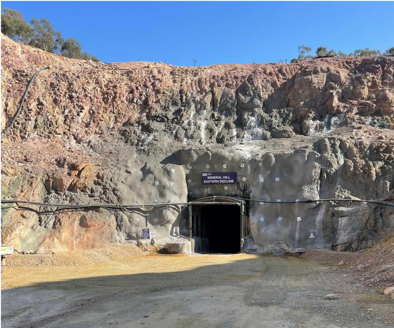
Figure 5: Rehabilitated Eastern Decline portal at Mineral Hill.
