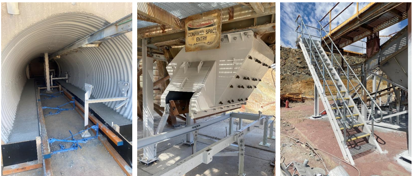
Figure 4: Mineral Hill plant - structural steel replacements and refurbished fine ore bin tunnels.
