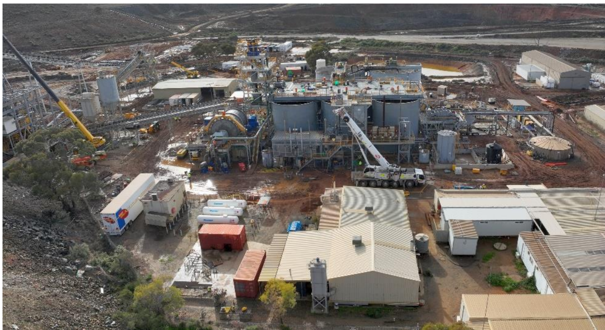
Figure 2: Three Mile Hill Mill refurbishment progress 29 June 2023
