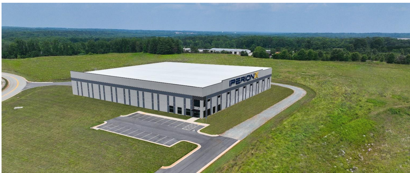
IperionX's permitted Titanium Production Facility in Virginia.
