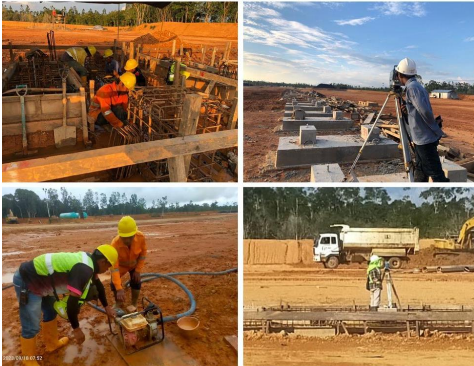
Batu Tuhup Jetty construction progress – piling works and foundation
