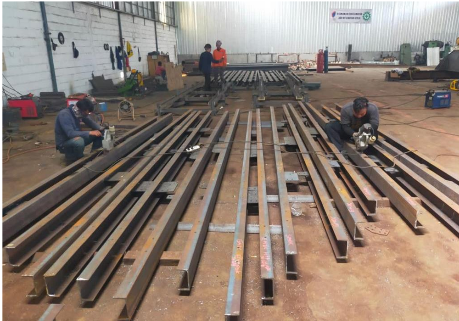
Structure fabrication progress for the conveying system
