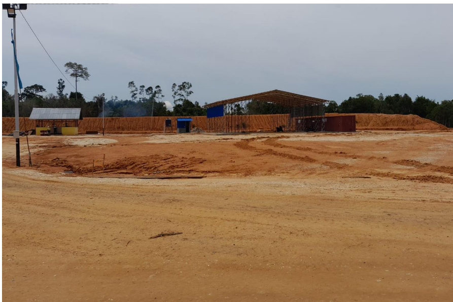
Workshop construction for coal trucks maintenance has been completed
