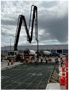
Figure 1. Concrete being replaced in full depth slab
