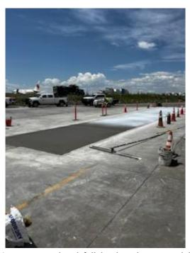
Figure 2. Completed full depth replacement slab
