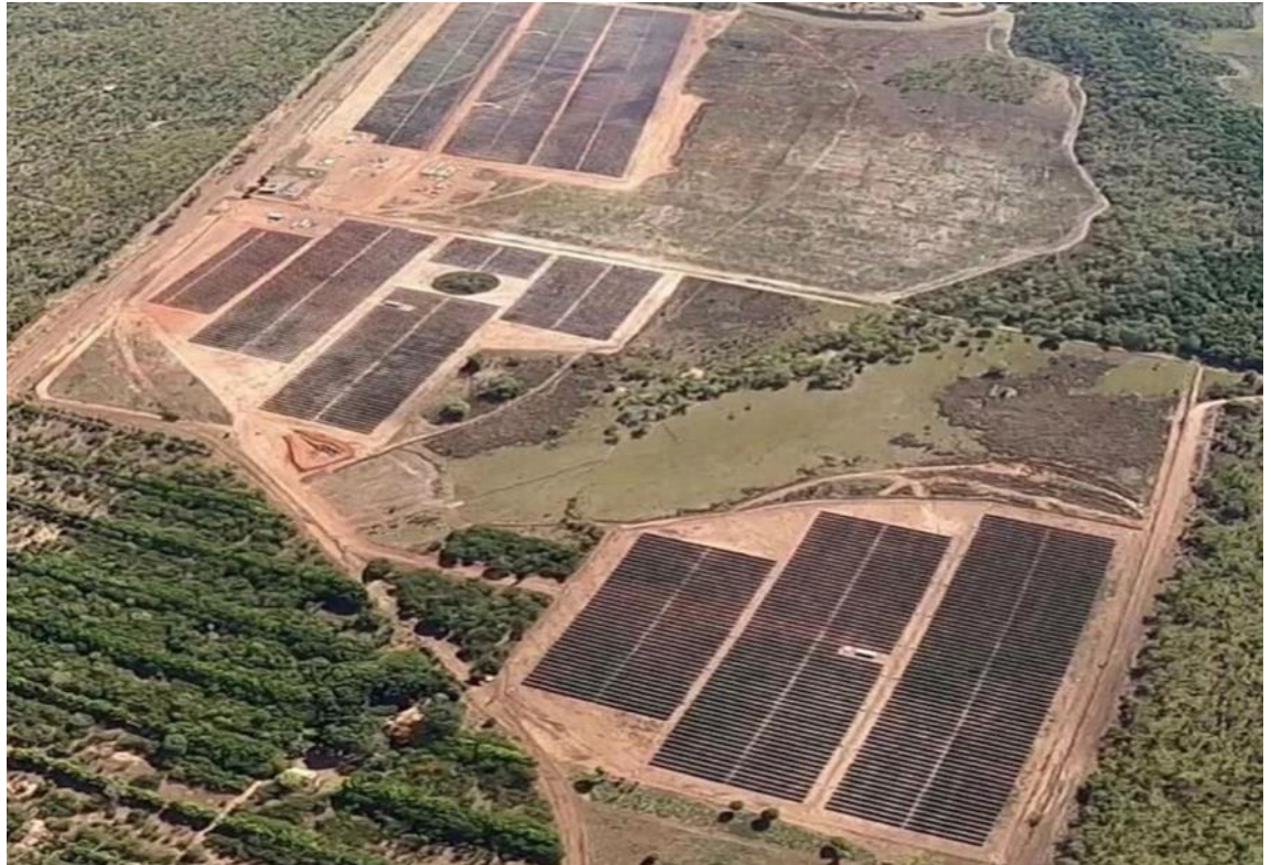
Figure 11 Solar farms at Batchelor (Batchelor 1 and Batchelor 2) adjacent to the Winchester Project.
