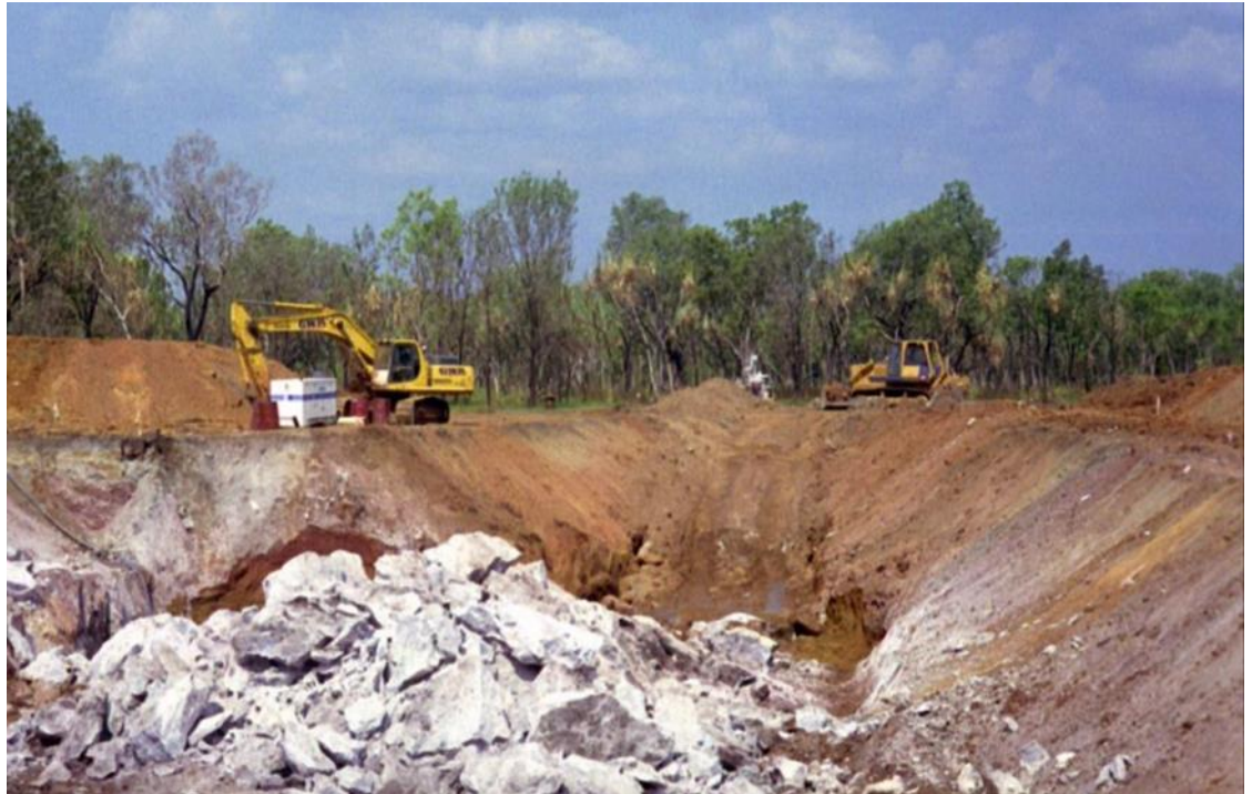
Figure 7 Test mining of magnesium at Winchester during the wet season (after blasting Level 0).
