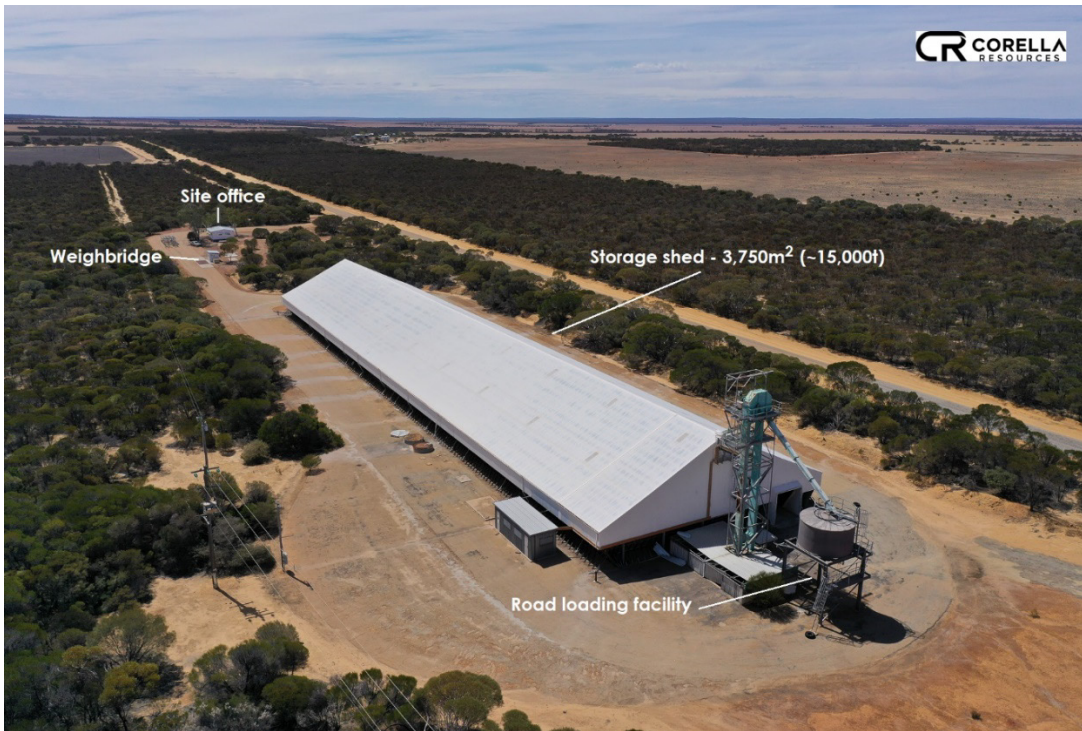
Figure 3: Tampu storage facility (view looking NNE)
