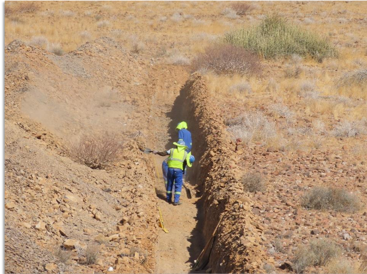
Figure 4: Clearing OP-T19 trench for sampling
