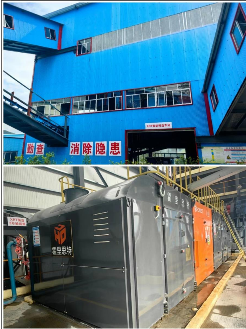
Figure 6-3: The Intelligent Preselection System plant
