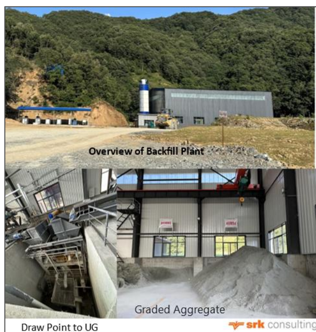
Figure 5-23: Backfill plant at LMW
