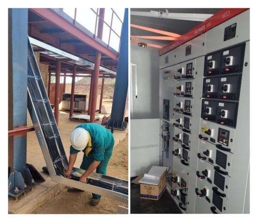
Figure 1: Installation of electrical cables within the cable racking (left) control panels within the Crushing MCC (right).
