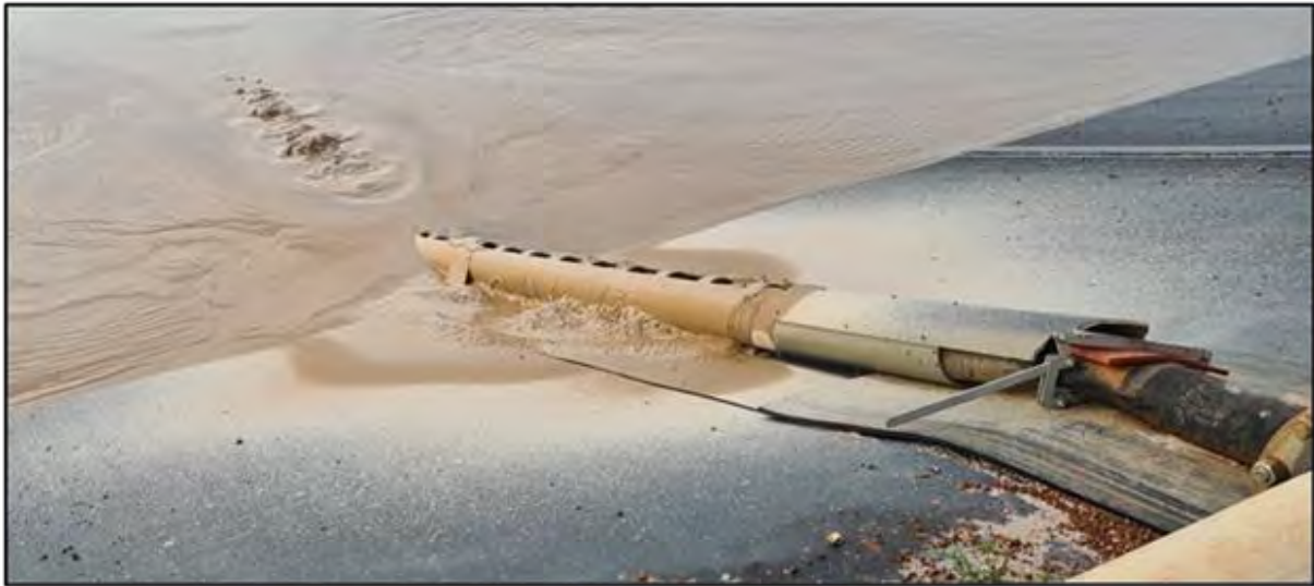
Figure 17-2: Conductor Pipe Detail on HDPE-lined TSF.
