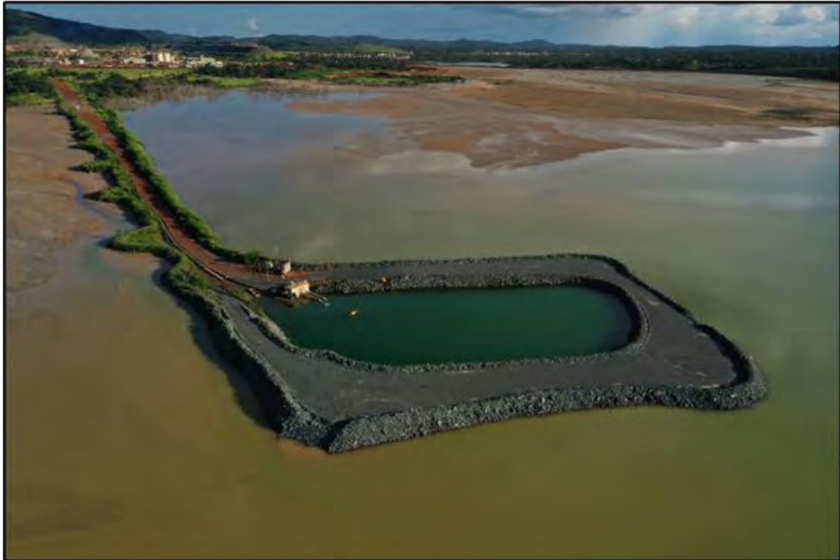
Figure 17-3: Decant Rock Filter.
