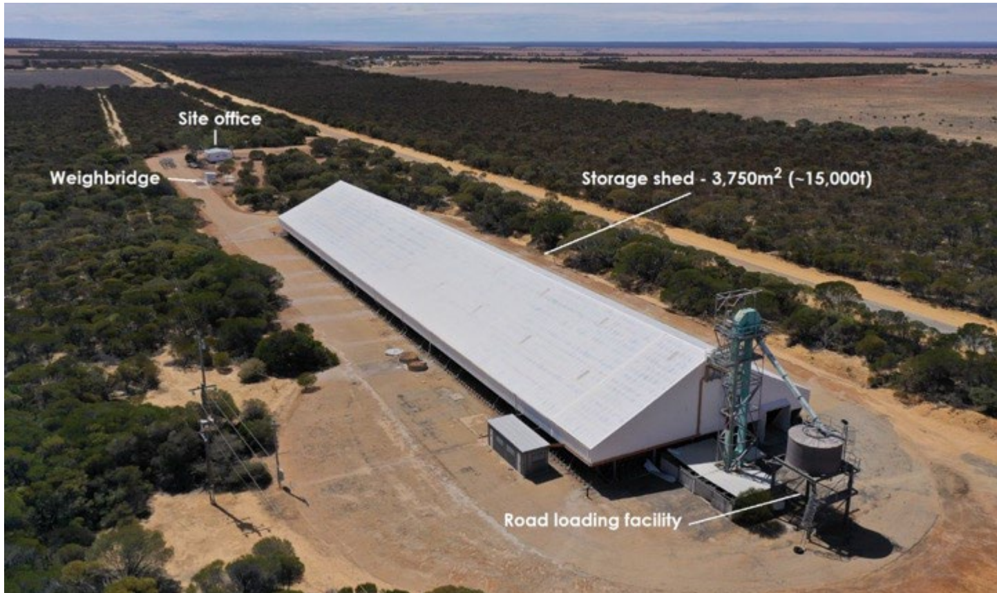
Tampu storage facility (view looking NNE)
