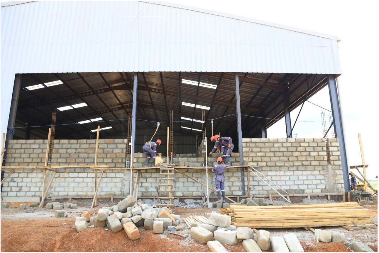
Figure 4: Construction of Technical Facility laboratory brickwork.
