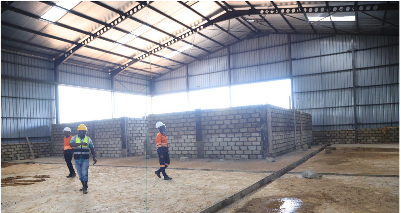
Figure 5: Technical Facility concrete slab, drains and sumps finalised and internal laboratory and office brickwork underway.
