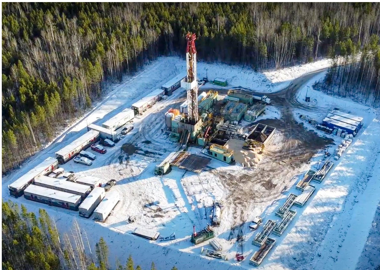
Figure 2. Gryphon Wapiti well site with drill rig.
